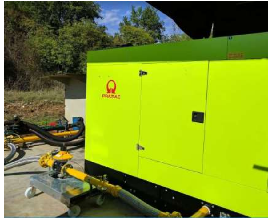
Factory Test of GGW400 Pressure rating: 25 mbar Load Steps: 0-50%-75%-90%-100%
